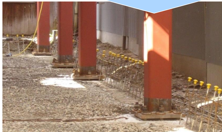
After construction work
