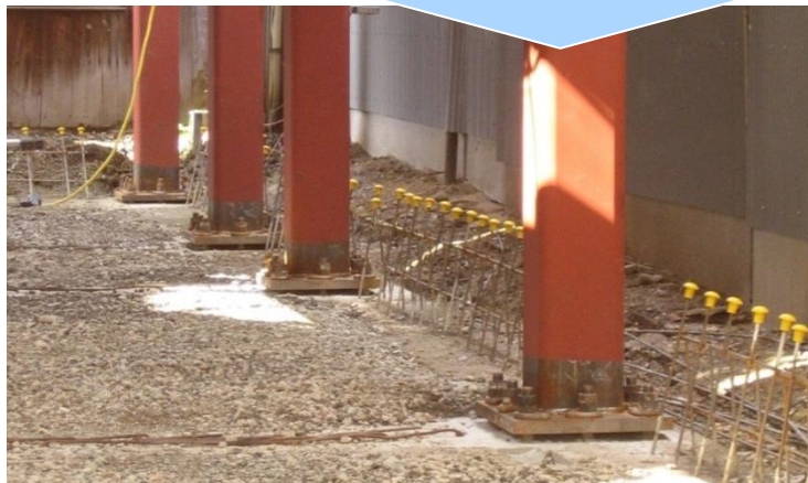
After construction work
