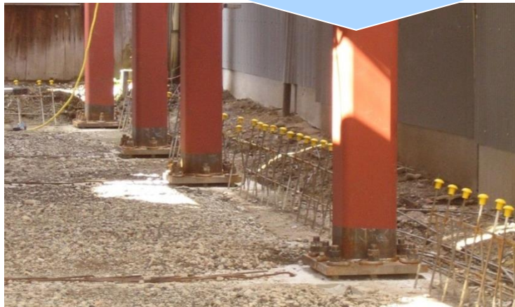
After construction work
