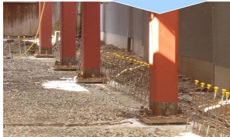
After construction work
