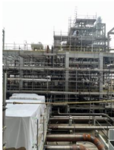
Biomass power plant construction site
