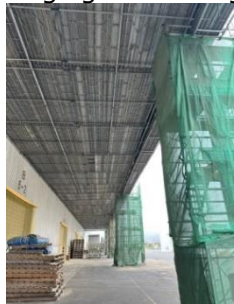
Wharf construction site (hanging scaffolding)
