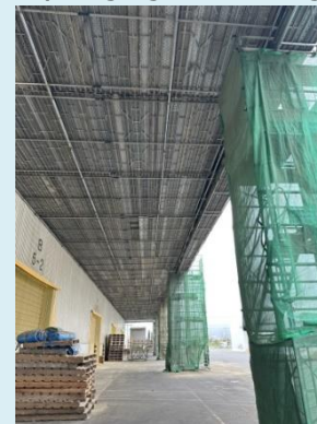
Wharf construction site (hanging scaffolding)
