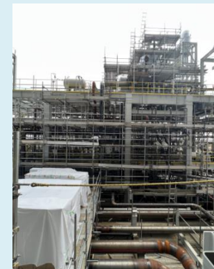
Biomass power plant construction site
