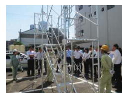
↑ Demonstration of assembly at the temporary construction materials training
