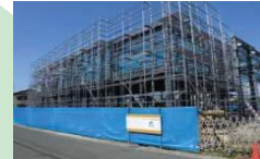
← Scaffolding construction services
