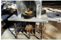
Steel frame foundation →
