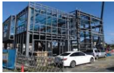
↑ Steel frame works
