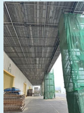
Wharf construction site (hanging scaffolding)
