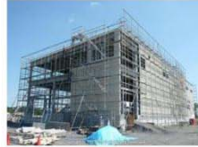
工場新築工事
